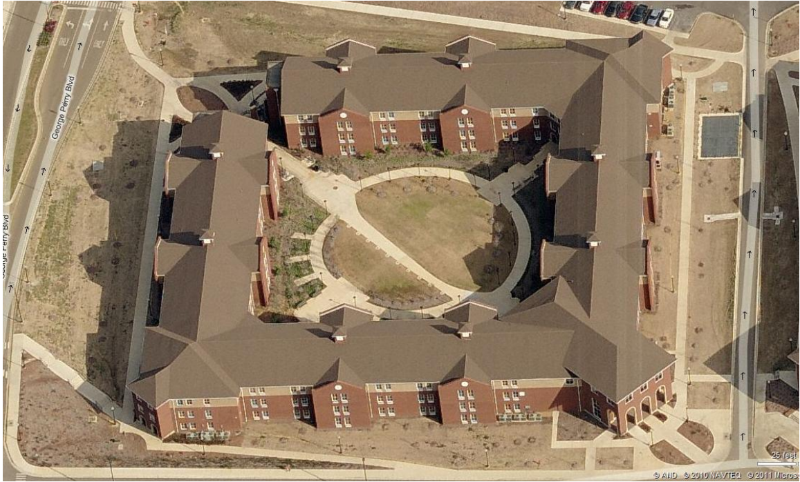
Figure 3.3 Birdseye view of the Ruby Courtyard. Source: Bing Maps.
