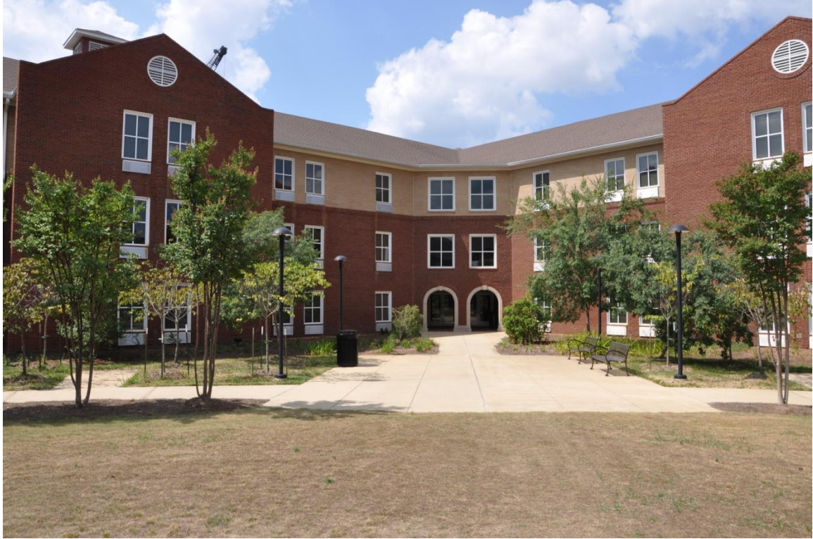
Figure 5.5 Image of the Ruby Courtyard showing how multiple light units are installed for a seating area. Source: Tariq Mahadin.
