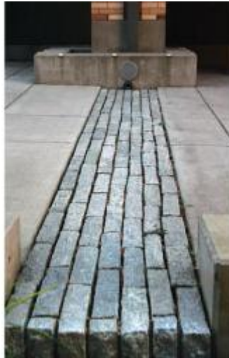
Figure 2.5 View of the rainwater trail from downspout to raised collection basin through scupper into granite-lined runnel. Source: Pennypacker 2008, 30.
