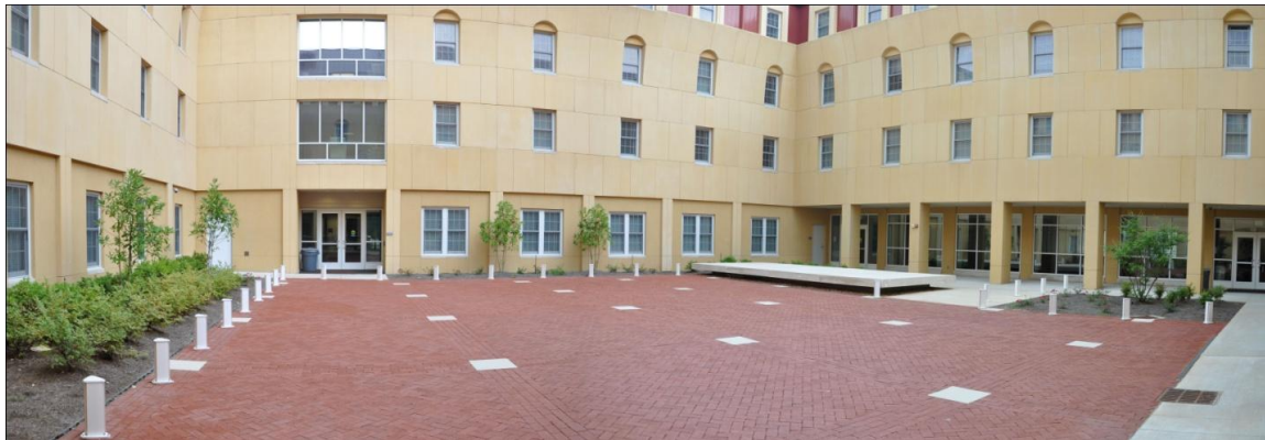
Figure 3.9 Panoramic view of the Residential Courtyard. Source: Tariq Mahadin.
